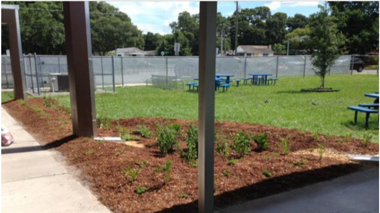
Figure 12: Bioretention BR 4 pre-construction (top) and post-construction (bottom)
