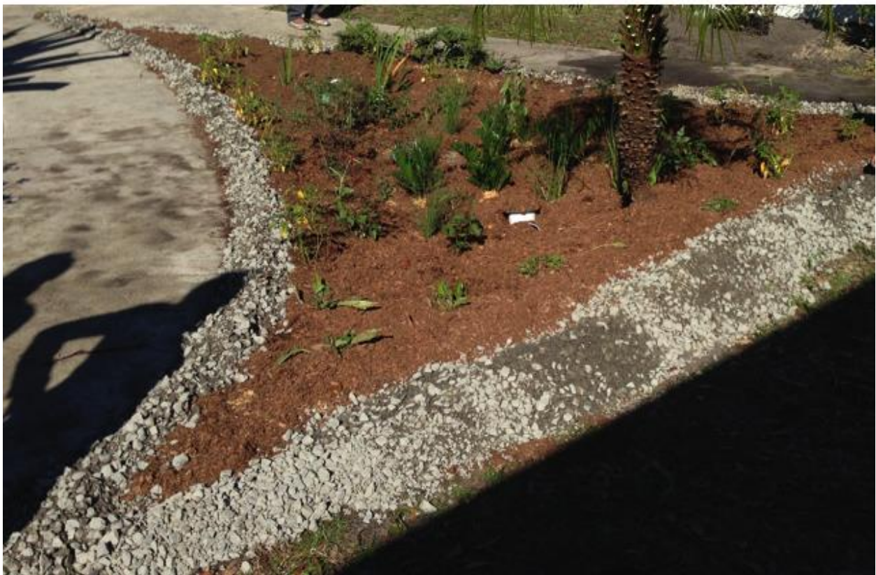
Figure 14: Bioretention BR 8 pre-construction (top) and post-construction (bottom)
